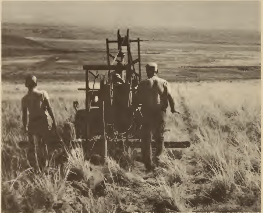
Figure 4.—Plastic pipe and machinery to lay it have allowed cattle to graze thousands of acres of previously unused western range. Here, tractor-drawn equipment trenches, lays, and buries plastic pipe at normal walking speed.
